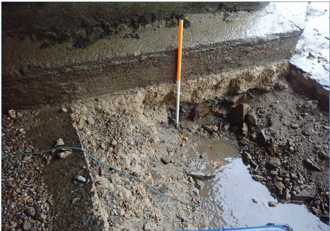
Plate 20: TP-03 at Pier 3, cleaned down as excavated.
