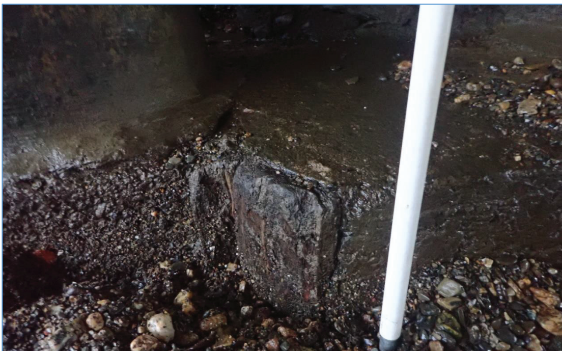
Plate 30: Pier 4, east facing side, showing a timber plank that survives as part of the form-work associated with the addition of the concrete surround to the stone piers, and which in turn is impacted on by the insertion of the concrete pile as part of the 1970s bridge-widening works.
