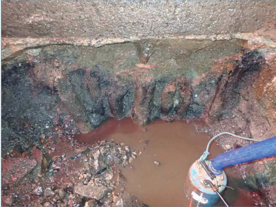
Plate 25: TP-04 at Pier 4. View of the fully excavated area.
