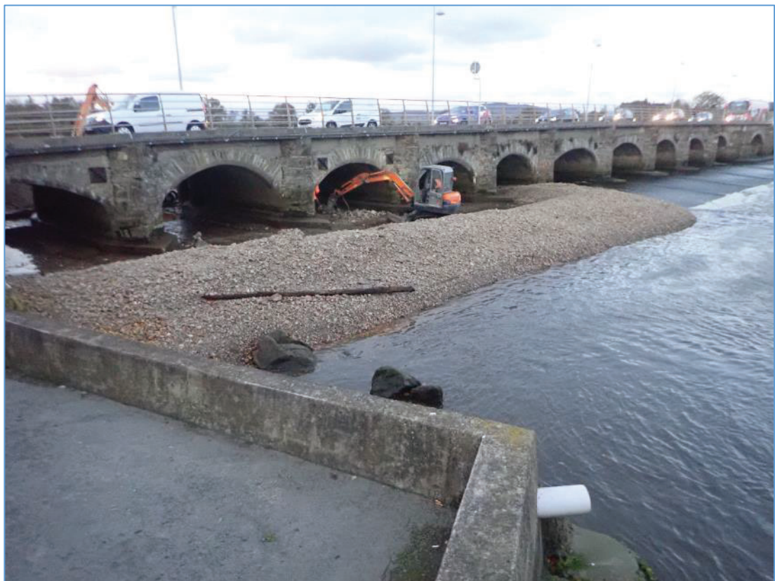
Plate 7: View from west bank of the bund created on the downstream side of the bridge.
