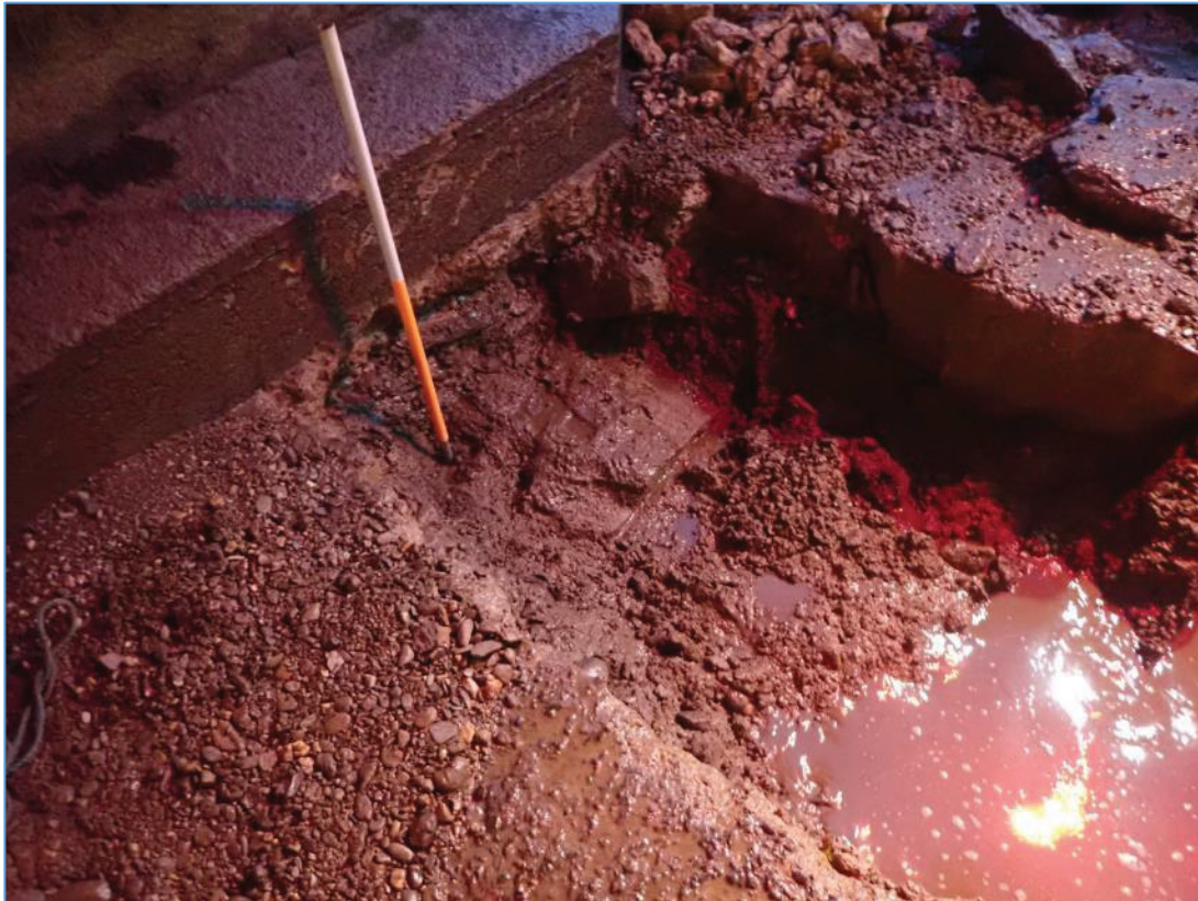
Plate 14: TP-02, view showing the full excavated depth at Pier 2.
