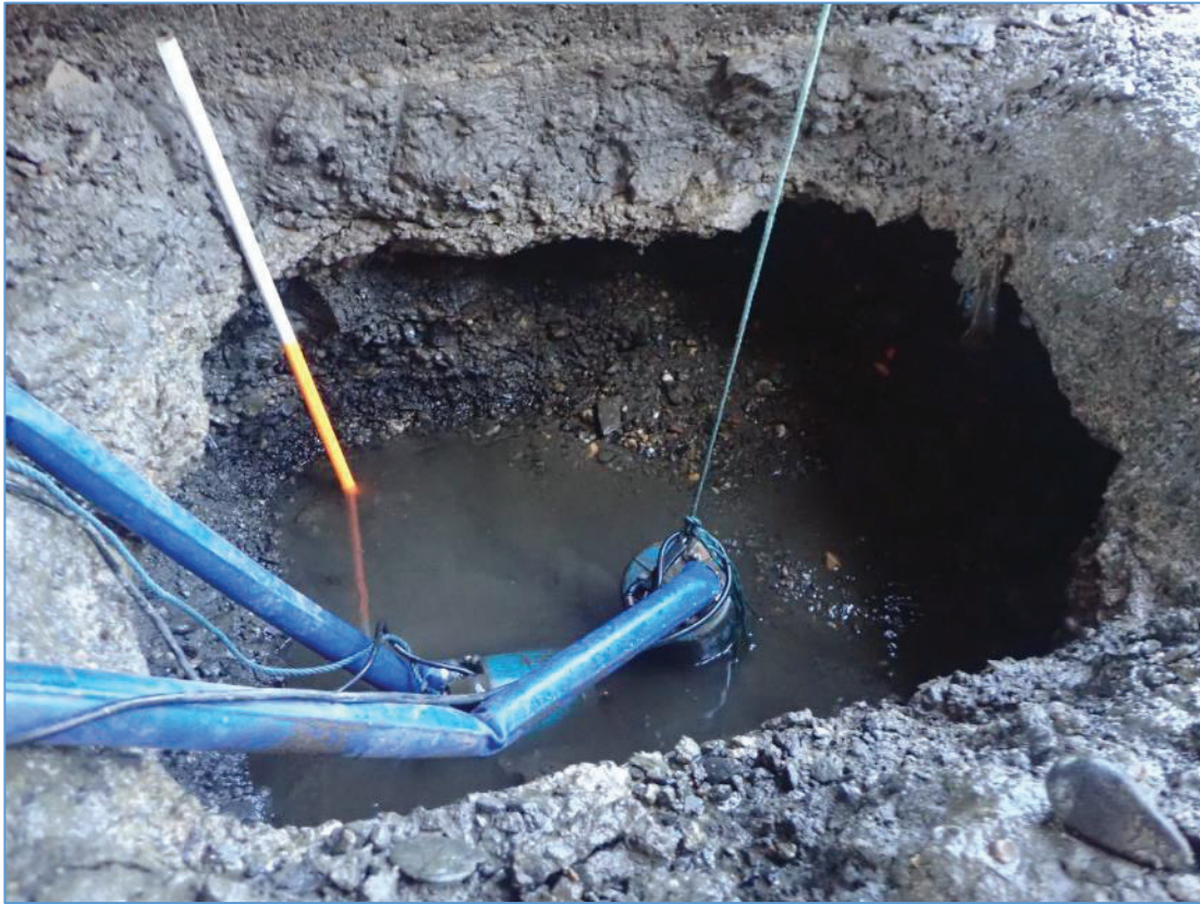
Plate 12: TP-01, close-up view showing large stone associated with the apron underlying the more recent concrete surface and overlying river shingle.
