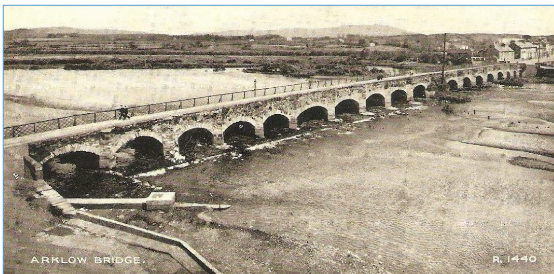
Plate 3: Historic photograph of Arklow Bridge taken from the west bank. Date unknown, Collection unknown. Source: ARUP.
